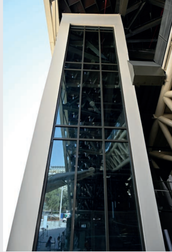
Republic of Korea Pavilion, Dubai, UAE E160 mullion/transom facade with fire protection and 15 degree incline – forster thermfix vario
