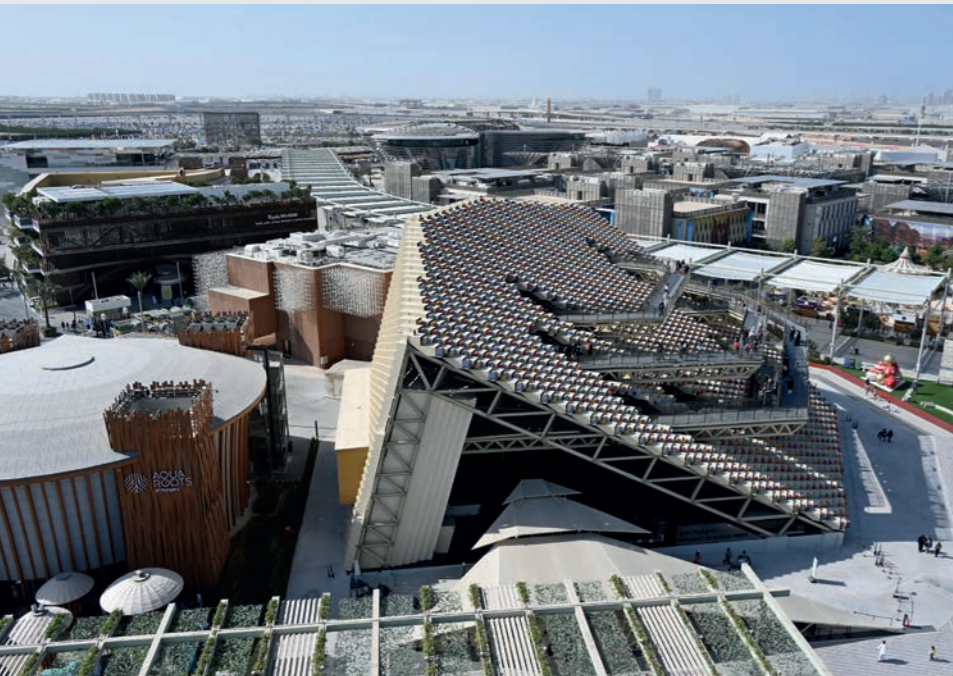
Republic of Korea Pavilion, Dubai, UAE E160 mullion/transom facade with fire protection and 15 degree incline – forster thermfix vario
