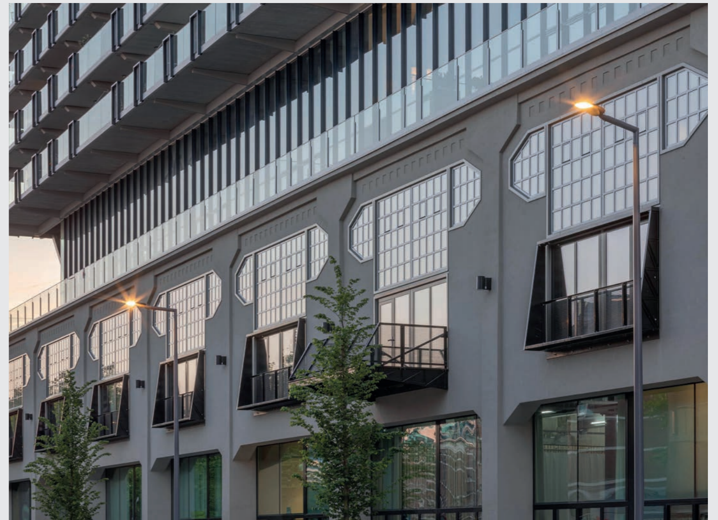
Fenix I, Rotterdam, the Netherlands Thermally insulated windows and fixed glazing – forster unico xs Image: Bart van Hoek Architectuurfotografie
